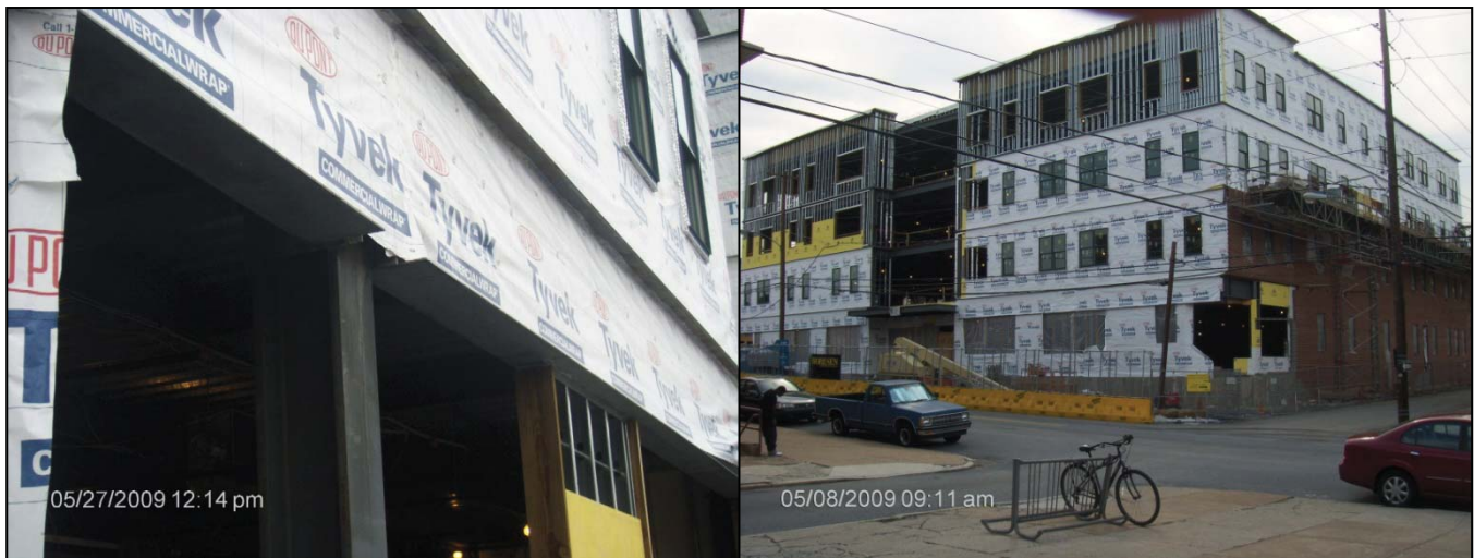
Figure 30 – Masonry Façade Steel Support Angles
